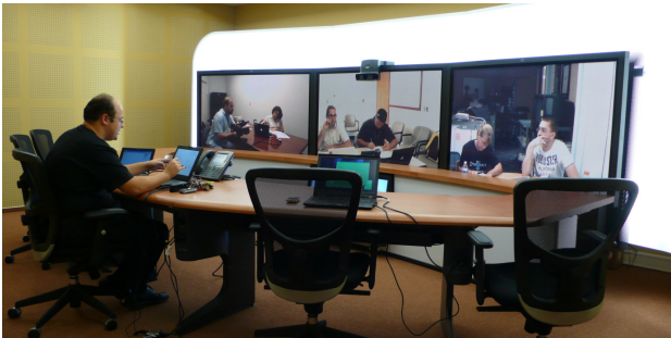
Figure 5. TUKE Cisco TelePresence unit
