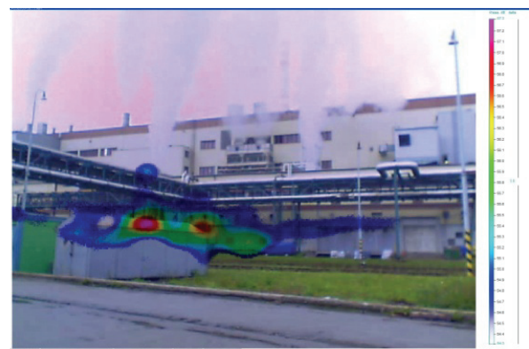
Figure 5. View of the analyzed buildings – 2 nd source
